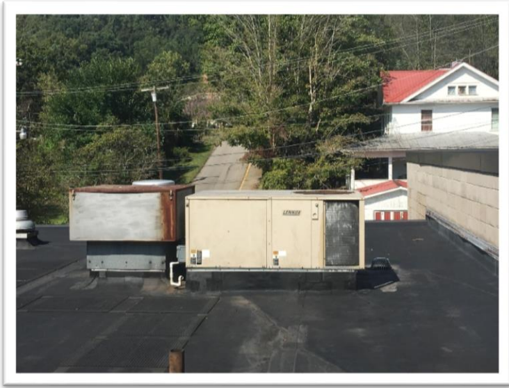
The antiquated rooftop equipment is proposed to be replaced at Sutton Elementary.
