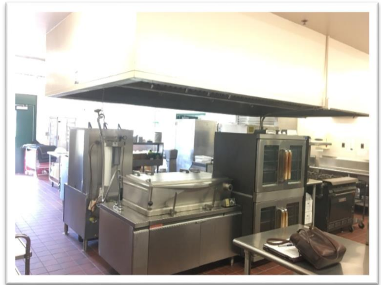
The county proposes to replace the existing kitchen hood at Braxton County High School.
