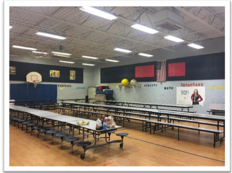
The dining and gym areas at Sutton Elementary lack proper air exchange capabilities.
