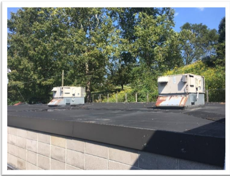
The antiquated rooftop equipment is proposed to be replaced above dining and gym at Sutton Elementary.
