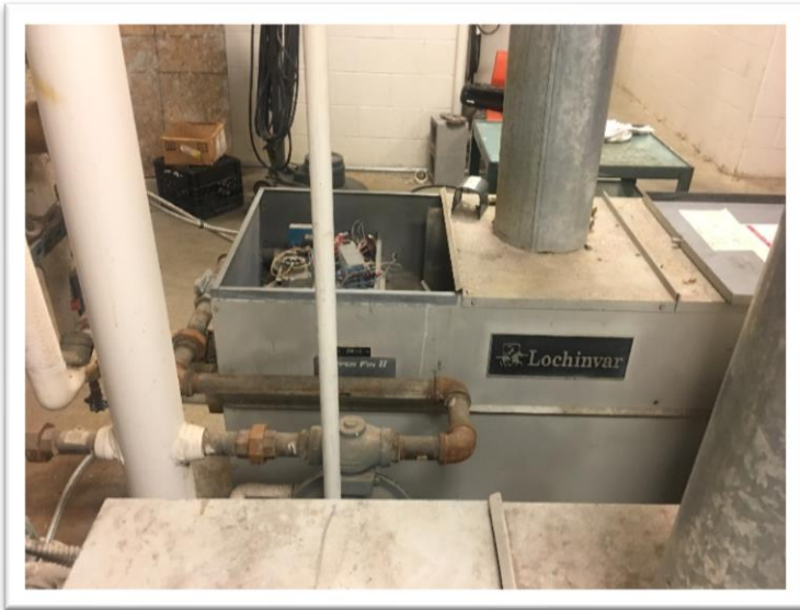
The existing equipment has reached the end of its life expectancy and replacement parts are difficult to find.
