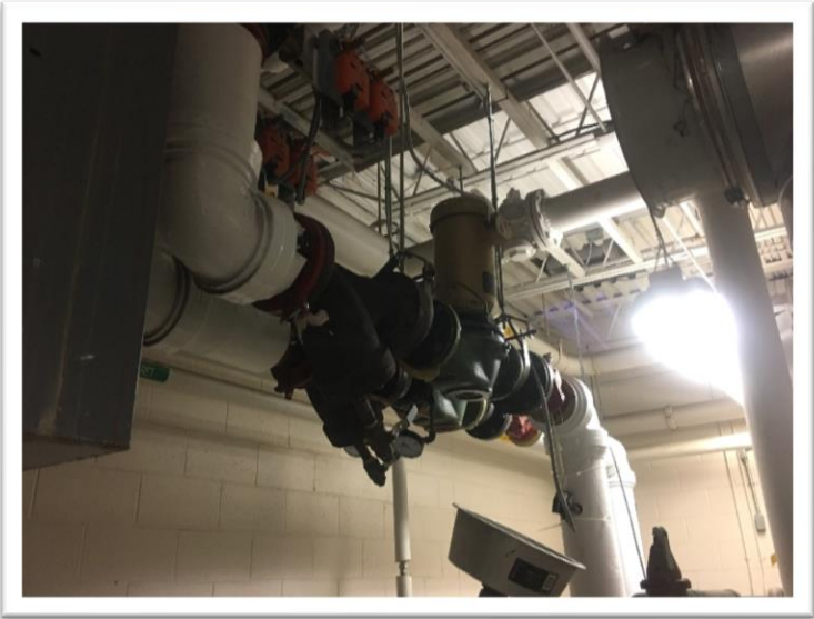
The existing pump leaks glycol and the maintenance staff catches the glycol into a barrel and refills the system.
