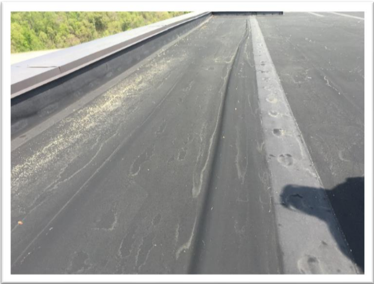
The roof is the original to this facility constructed in 1998. Overtime, water has entered the classroom spaces during rainy day.
