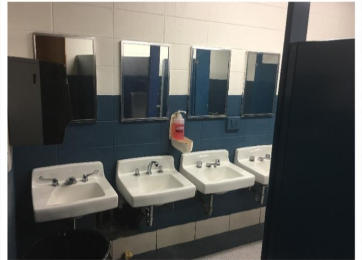
The existing restrooms do not meet ADA requirements. Renovations will bring restrooms up to current code.
