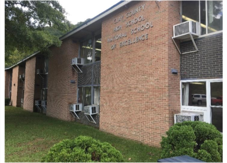
Existing widow air conditioning and wall heaters will be replaced with a New HVAC system throughout facility.
