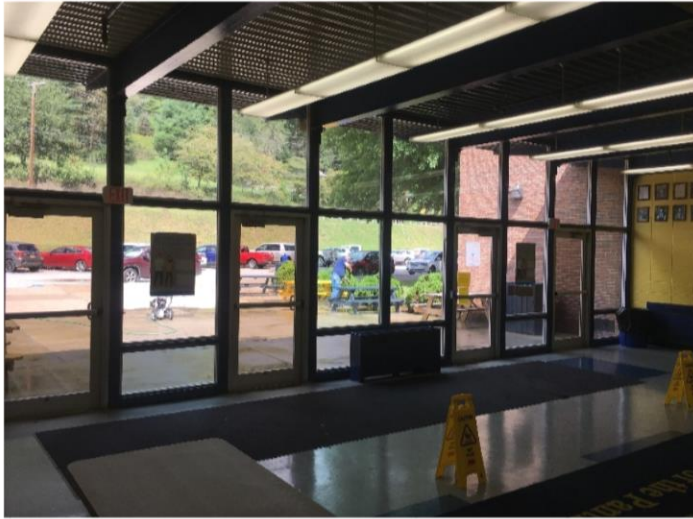
The existing main entrance is unsecure and allows direct access to the main hallway.
