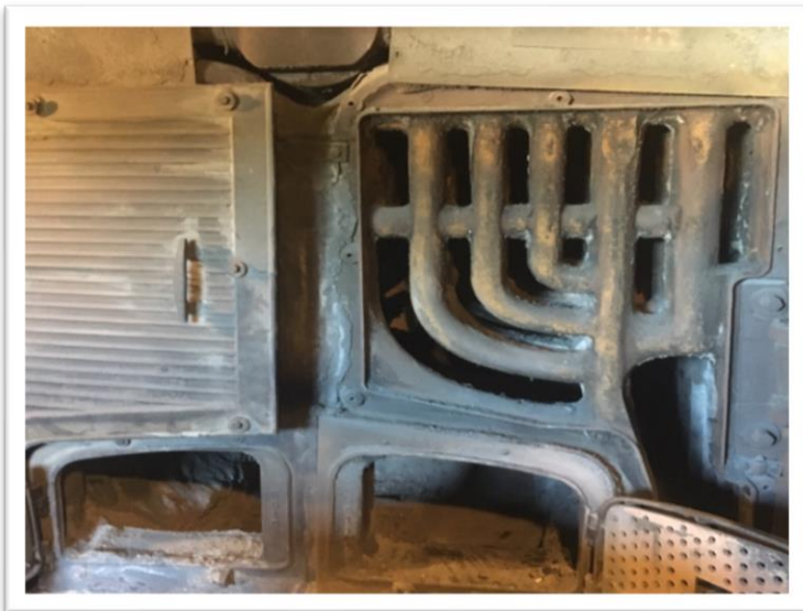
This is the coal fired boiler used to heat the High School facility. The custodial staff must fill the hoppers from the coal bin every 2 hours in order to keep the school at a reasonable temperature during cold weather.
