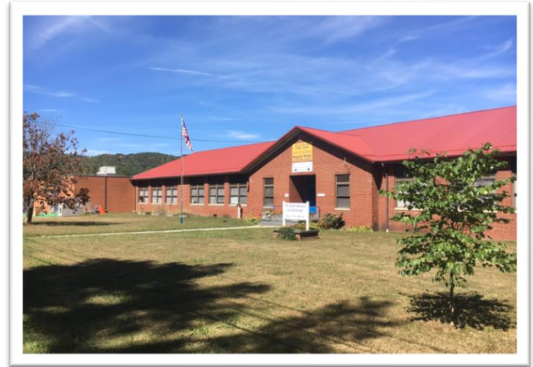
The front entrances to both Meadow Bridge High School and Elementary School do not have separate, secure visitor entry points.
