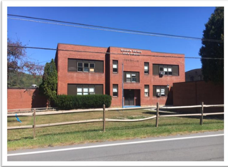
In addition to the life, health, and safety issues at Meadow Bridge High School, the building's 2 nd floor has been condemned since 2015.
