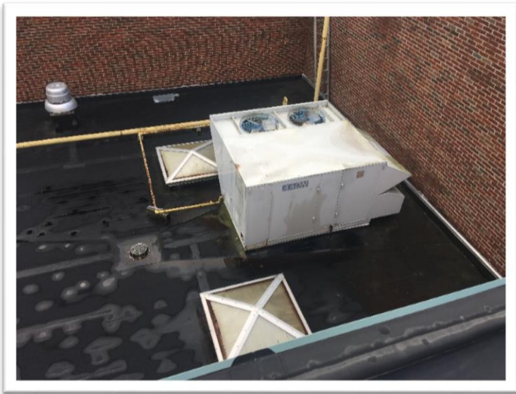
This is a roof top unit to be replaced over the weight room.
