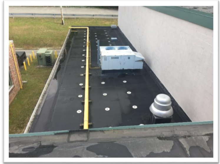
Image of a roof top unit to be replaced over the locker rooms.
