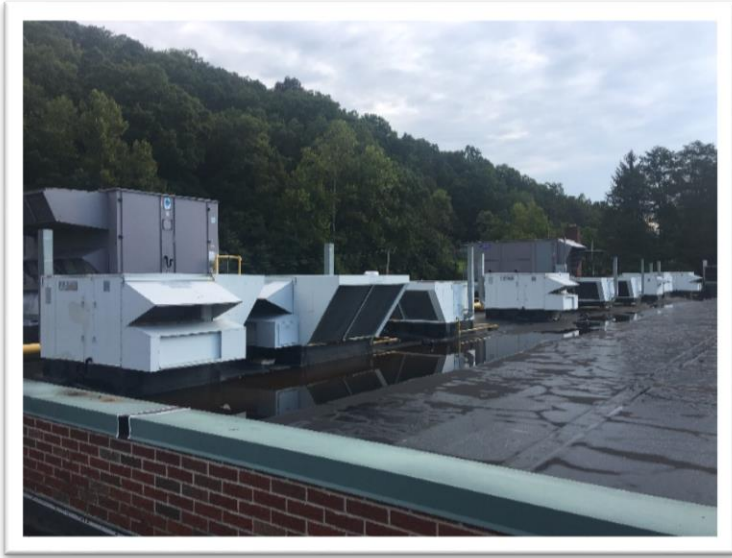
The existing roof top units do not provide adequate air exchange.
