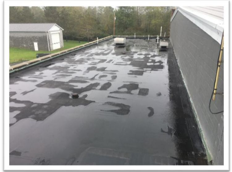
The existing roof has low spots and allows standing water. Leaks are found throughout the facility causing damage ceiling tile.
