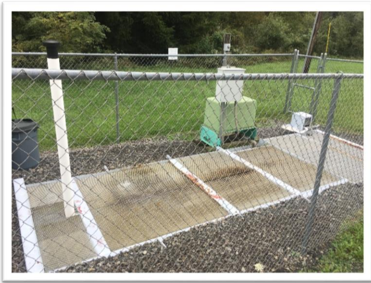
The existing water treatment plant is over forty years old and multiple leaks due to rusting equipment.
