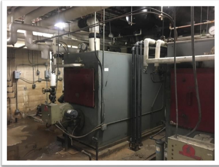
The existing boilers are fifty years old and have outlived their life expectancy.
