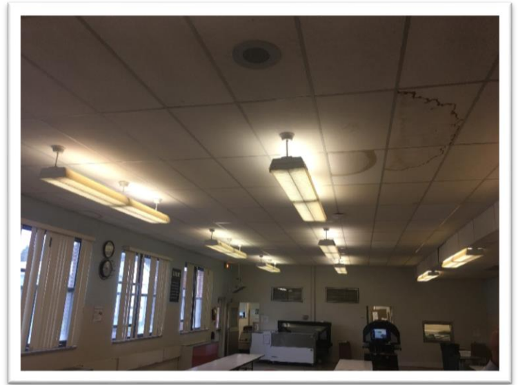
The existing lighting is outdated and inefficient. Ceilings are old and damaged from leaks in the roof.
