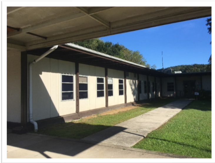
Wilsonburg Elementary was a modular structure that has been use beyond its intended life expectancy.
