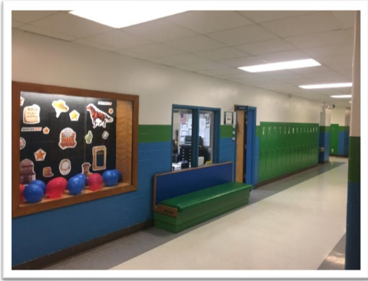
The current main entry allows visitors to have access to the entire facility prior to reporting to the main office.
