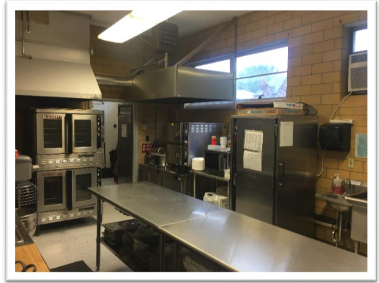
The existing kitchen is extremely undersized and inadequate for this facility.
