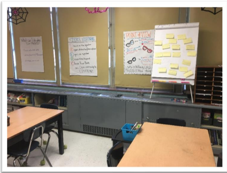
The existing wall units are inefficient and have reach the end of its life expectancy.
