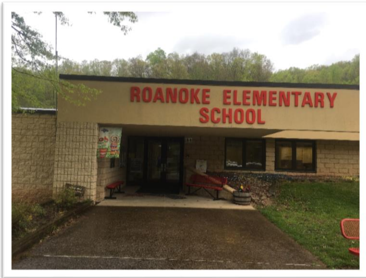
A new safe school entry will be constructed at Roanoke Elementary School to provide controlled visitor's access directly to the main office.
