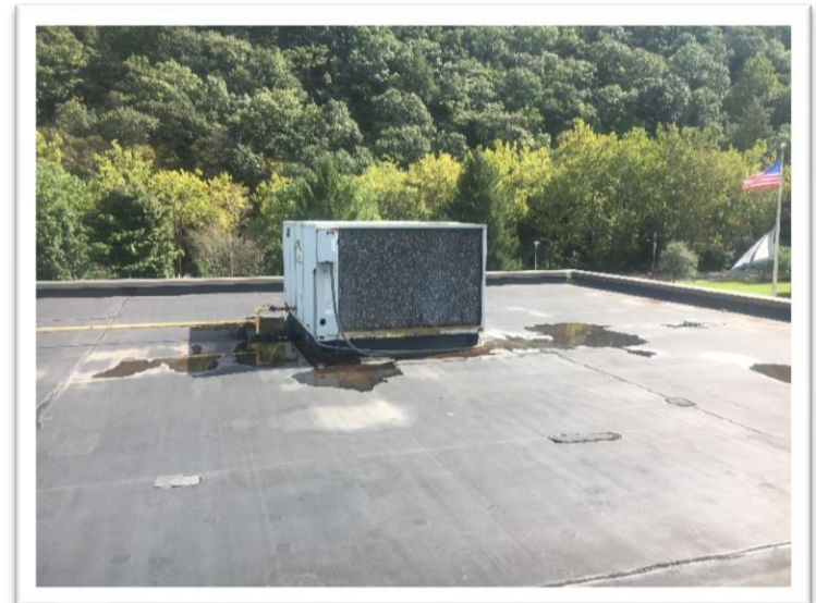
Typical roof top unit and example of ponding water on the roof of Keyser Middle School
