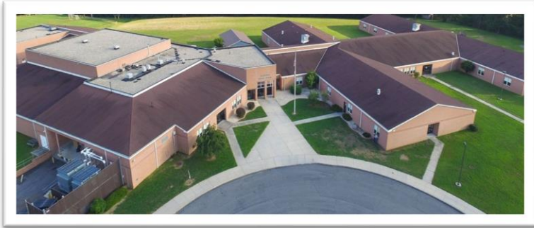
Overview of the Frankfort Middle School facility and roofing area.
