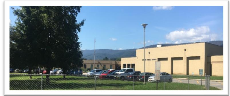
Bus loop/ parent drop of area and front entry view of Keyser Middle School
