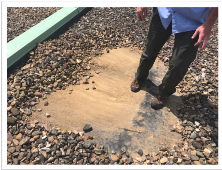
In certain areas the insulation and deck have sunk, and water does not drain correctly.
