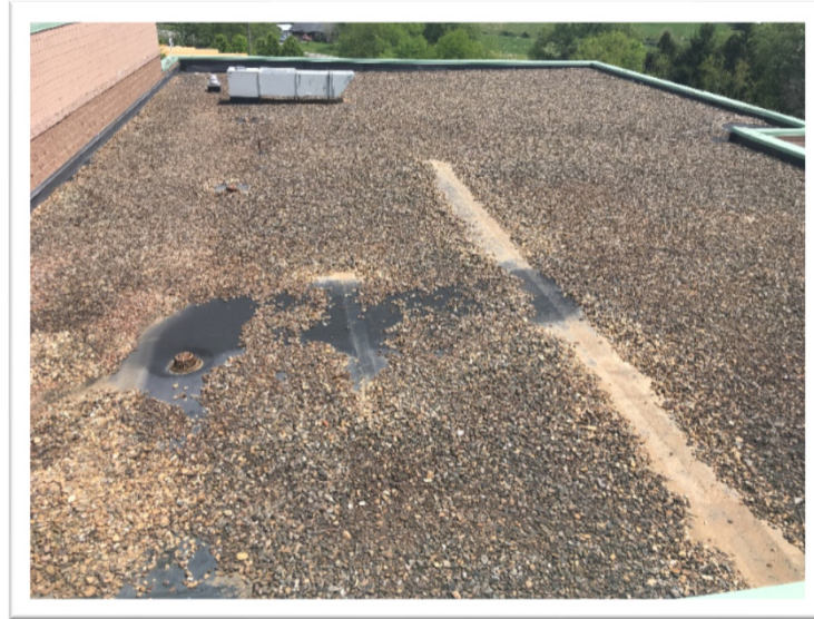
Maintenance staff must remove gravel to find leaks.
