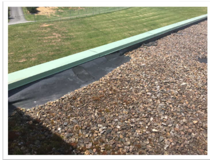
Bridging has occurred here, which is when the membrane no longer adheres to the parapet and pulls away from the wall.
