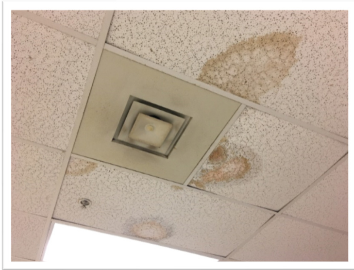
Leaks staining the ceiling tile is a common occurrence throughout the facility.
