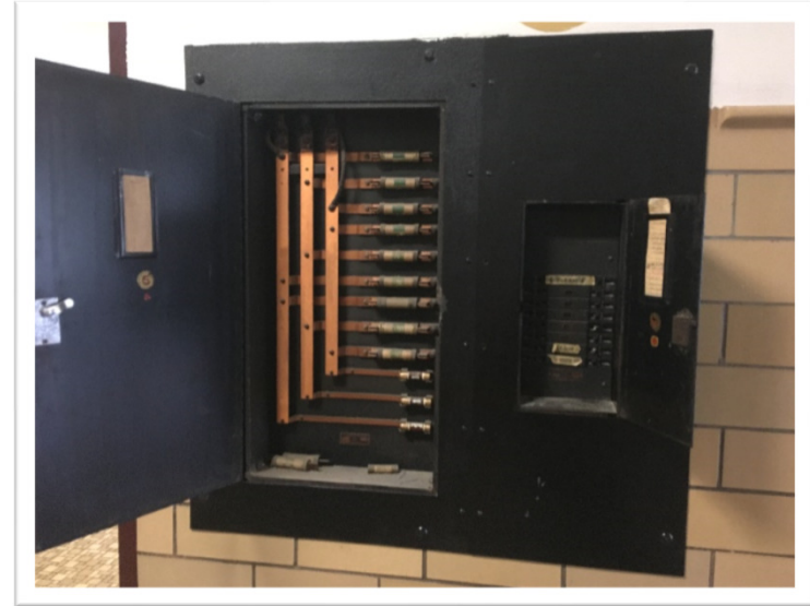
The project proposes electrical upgrades including the electrical panels that still have fuses.
