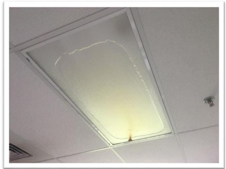
There is water in light fixtures from where the roof leaks. Damaged ceiling tile is present throughout entire Pendleton MS/HS facility.
