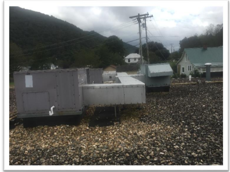
North Fork Elementary School's HVAC units are original and have outlived their life expectancy.
