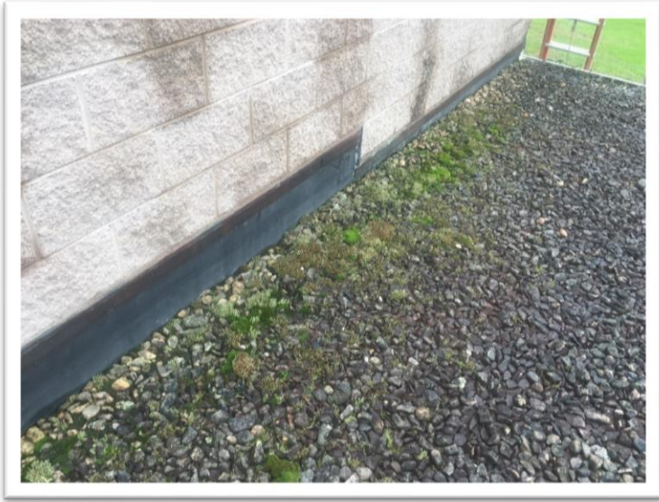
North Fork Elementary School has moss growing on roof due to standing water.
