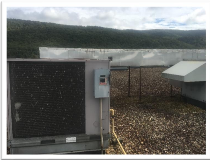
The existing HVAC units have outlived their life expectancy and are insufficient at Pendleton Co. Middle/High School.
