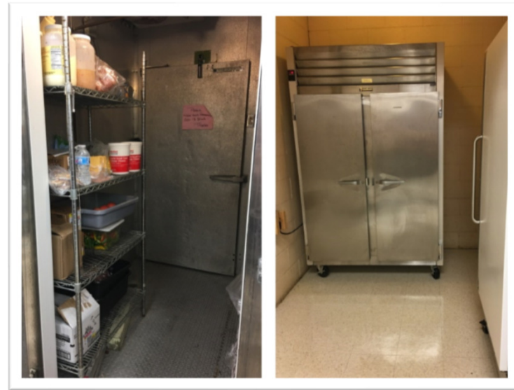
At the middle school, staff must pass through the cooler to get to the freezer. There is a storage room available for expansion nearby.
