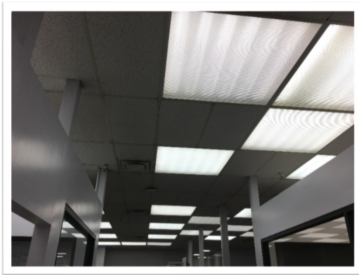
At Pleasants County Middle School, some areas of lighting are a 4'x4', which is a non-standard type and difficult to replace.
