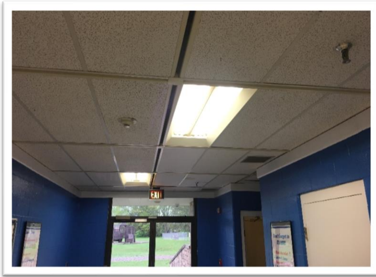
The existing lighting is original to these facilities that were constructed in the mid 1970's.
