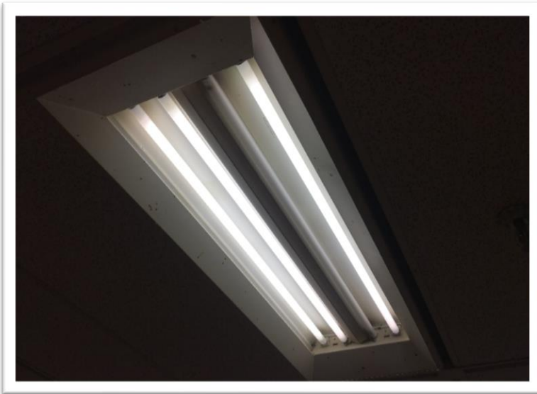
The existing lighting fixtures are unique sizes and maintenance staff has trouble finding replacement bulbs.
