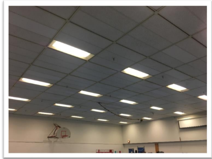
The lighting in multipurpose spaces are unprotected and creates safety concerns during physical education activities.
