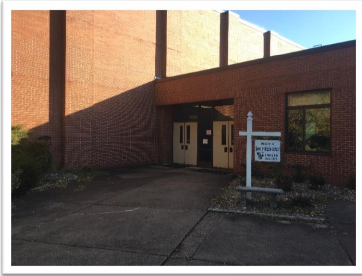
The main entrance of Spencer Middle School is not ADA accessible and is not adjacent to the office.
