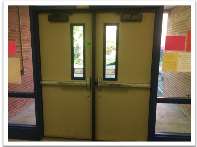
There are many unsecure and uncontrolled entrances that allow direct access to hallways.
