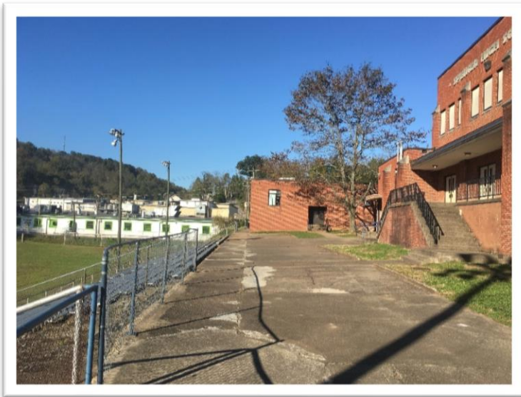
Many areas of the existing school have been condemned including the 3 rd and 4 th floors and a large section of bleachers.
