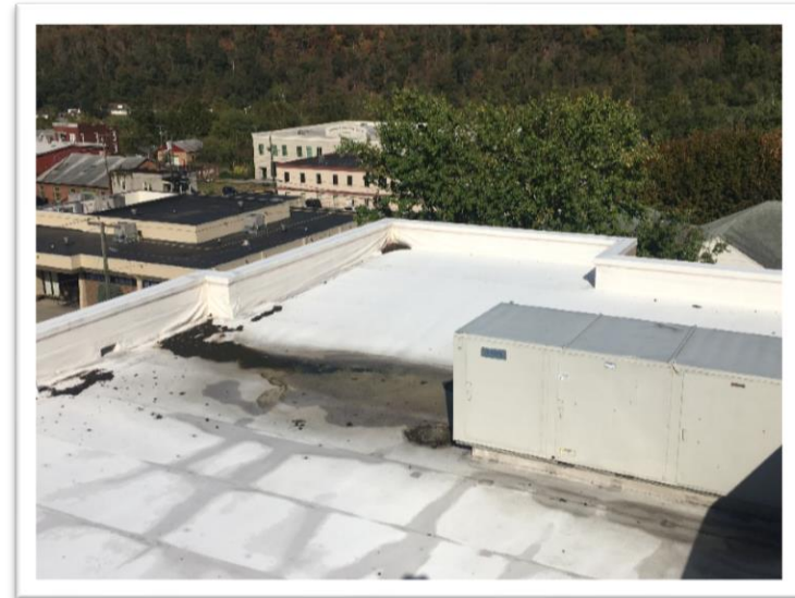
Ponding water and failing wall flashings in the Thermoplastic roofing. This area can not be patched due to the type of roofing membrane used.
