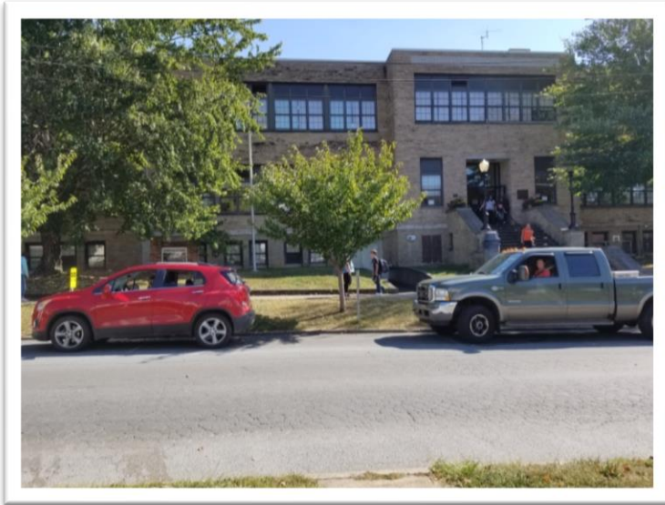
Street view of Summers County MS showing mold stains from moisture issues both above and below the windows. This is typical throughout the facility.
