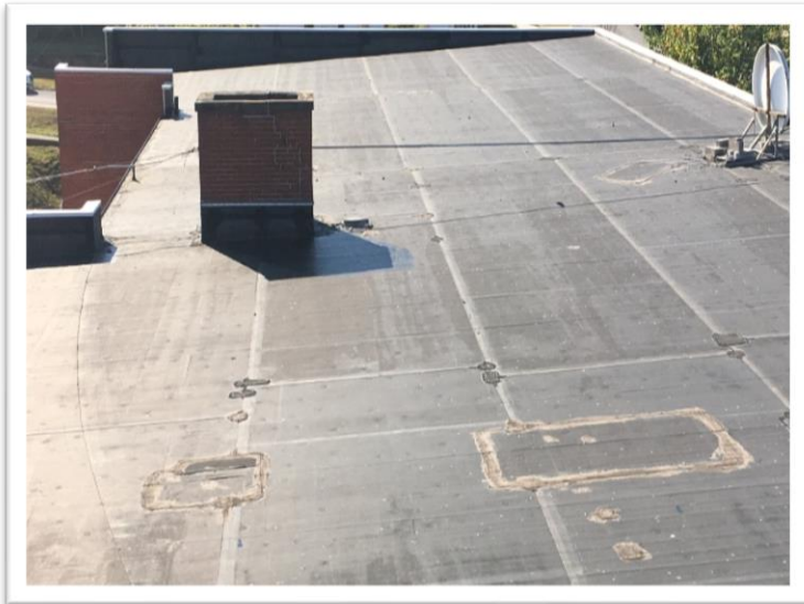
Example of the extensive patching and repairs performed to the EPDM roofing by the county maintenance staff in an attempt to slow roofing leaks.
