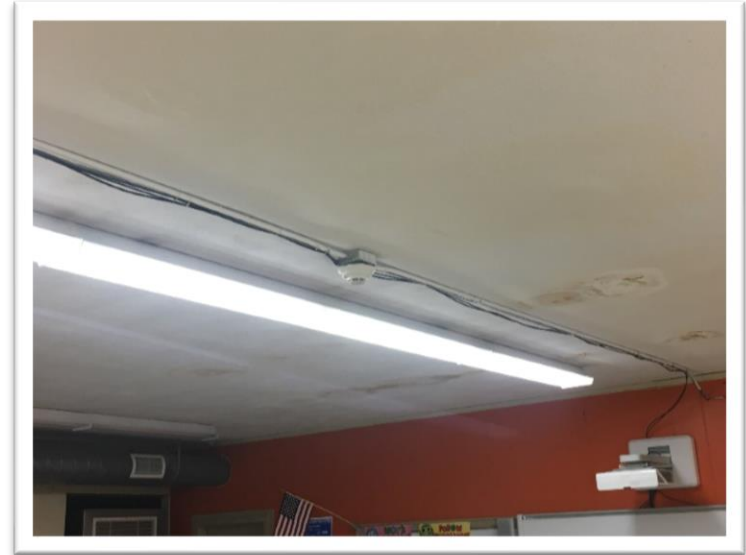
Roof leaks are common throughout the facility and cause regular disruptions to the students during rain events.
