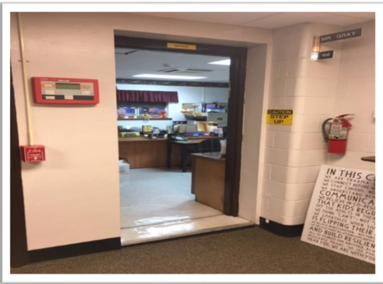
The existing office is small and inadequate for this facility. An existing classroom will be renovated to create a new main office area.
