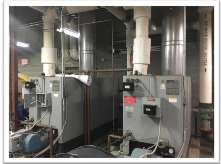
The existing boilers will be removed as they will not be needed with the new system.
