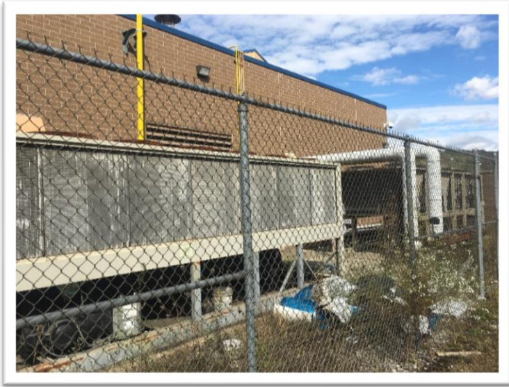
The existing chiller system will be removed and replaced with rooftop units at this facility.
