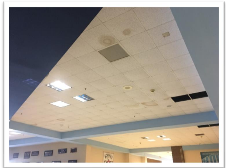
The existing damaged ceilings will be replaced after demo of the existing HVAC system.
