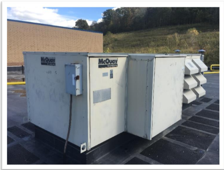
The remaining existing rooftop units will be replaced with a new efficient rooftop units.
