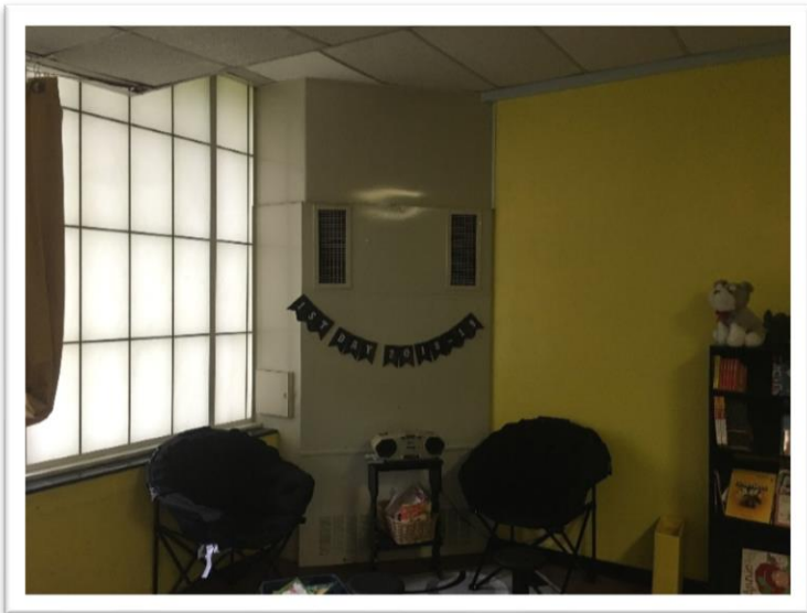
The existing HVAC units have reached the end of its life expectancy. New HVAC will provide a quieter, safer, and healthier environment for this facility.
