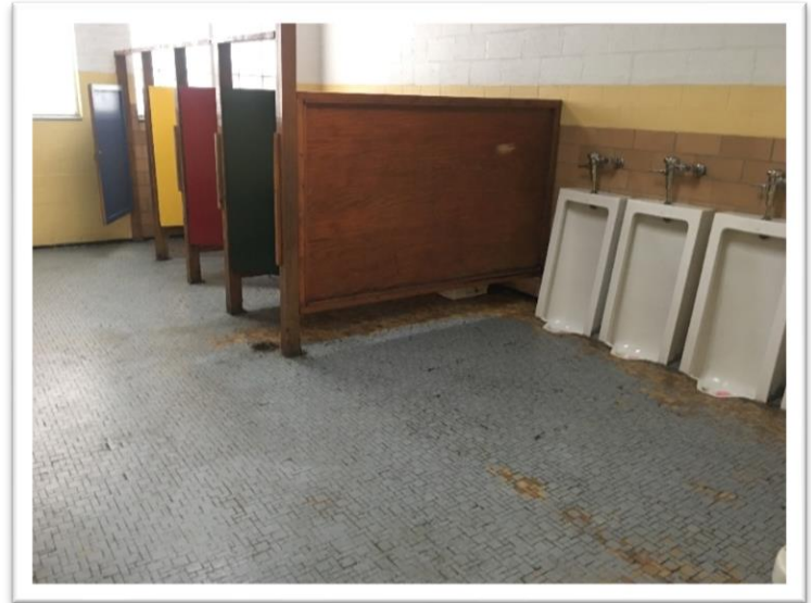
The existing restrooms will be renovated to meet current ADA standards.
