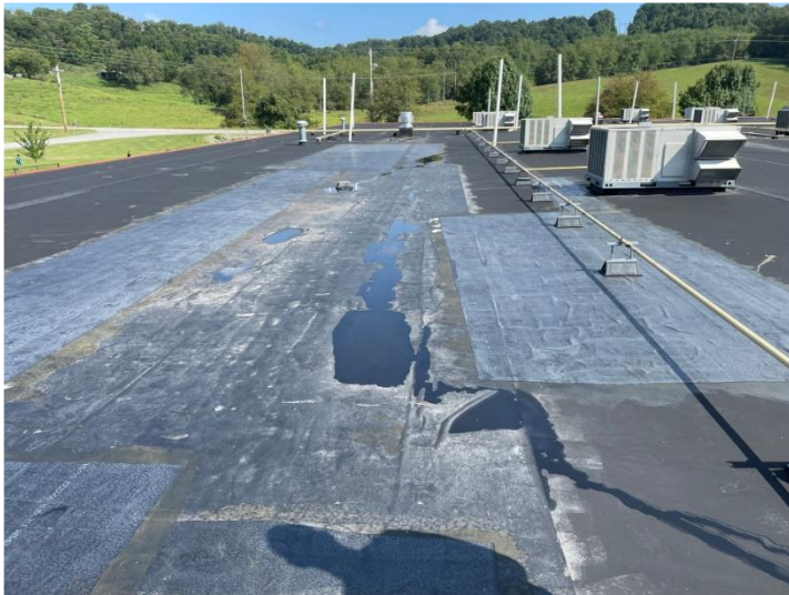
Large patches on roof to fix leaks.
