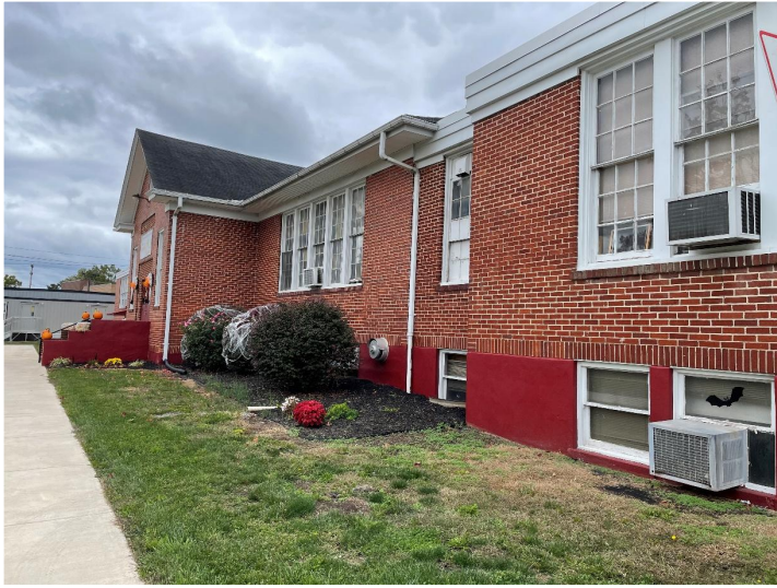
Front of current Inwood Primary to be demolished and new (PreK only) facility to be built on site.
