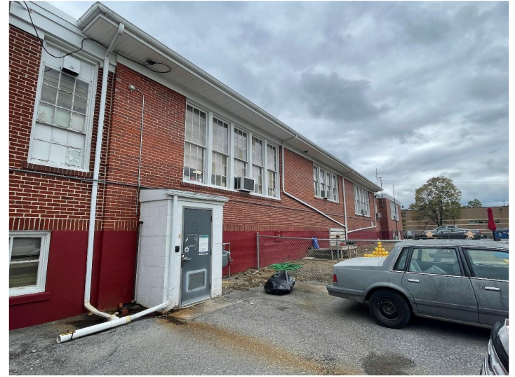
Rear of current Inwood Primary to be demolished and new (PreK only) facility to be built on site.
