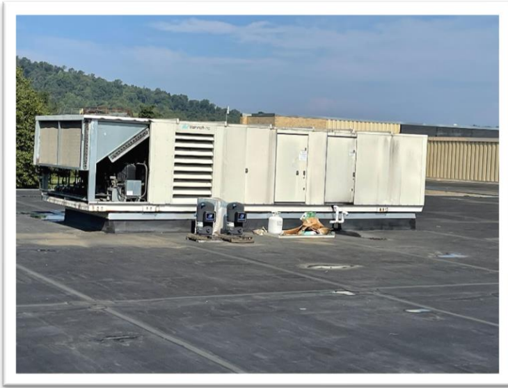
Mammoth Roof top unit showing ongoing replacement of compressors. Replacement parts are becoming obsolete.
