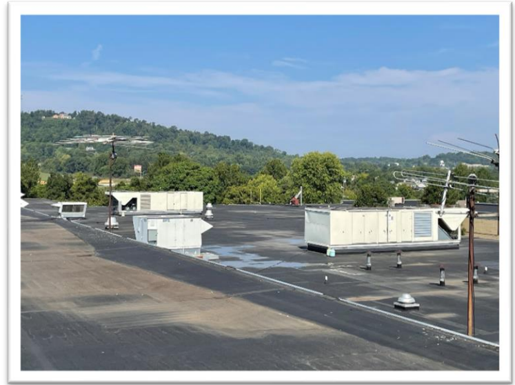
Roof replacement is proposed over this portion of the facility. Ponding occurs as slopes fail.
