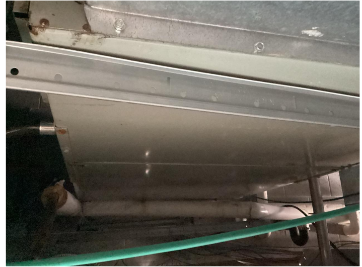
The HVAC units are original to the building, are located above the ceiling, and need constant repairs.
