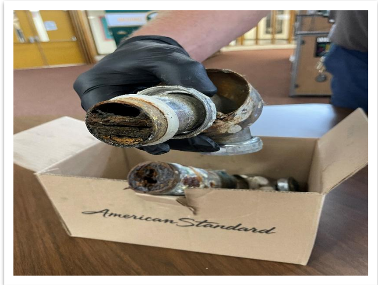
Existing pipes are over ½ way clogged, which obstructs camera from videoing the entire piping system.
