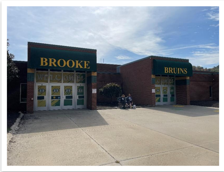
Brooke County High School was built in 1967, original piping is deteriorating and creating major issues at the facility.
