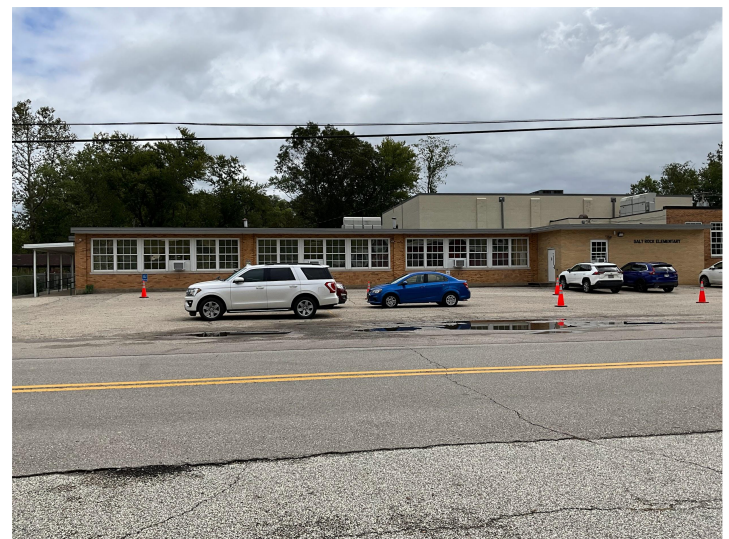
The facility has no fire sprinkler system. The Salt Rock Fire Department is ~500' from the school.
