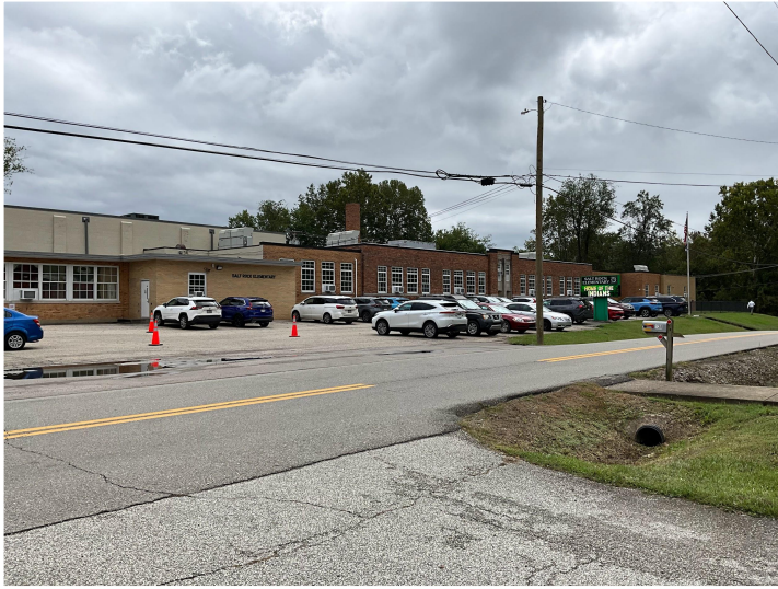
The facility was funded by the SBA for a new HVAC system in 2013. That system has surpassed its 10-year life expectancy.
