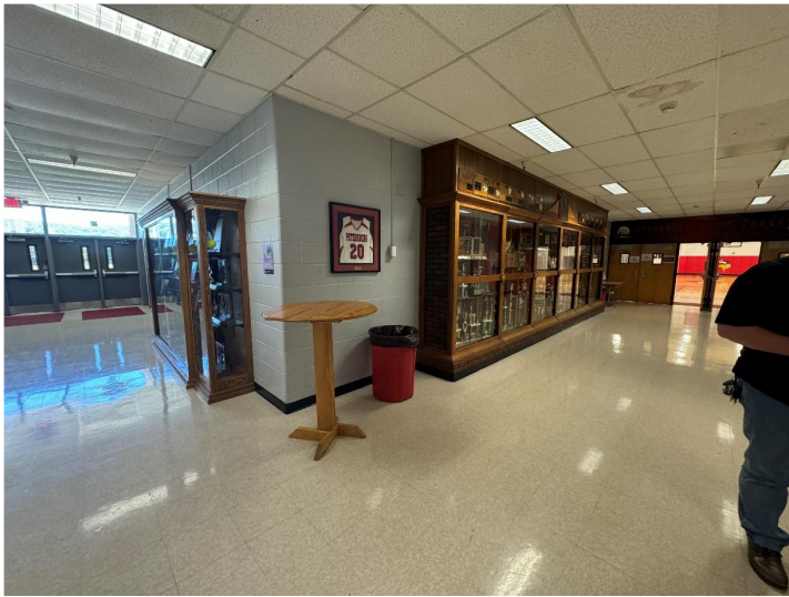
Doors on the left will be the new entry point closer to the gymnasium and cafeteria which are used after hours.
