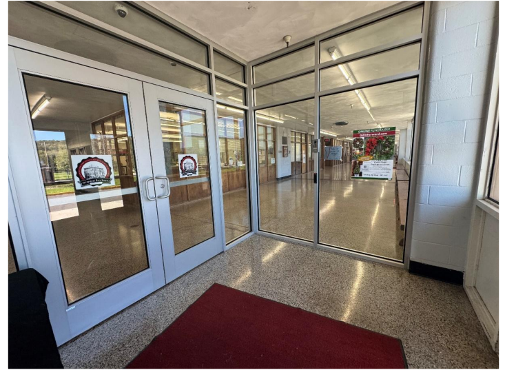
Current vestibule with main office across the hall. This office will become a wellness suite for the school.
