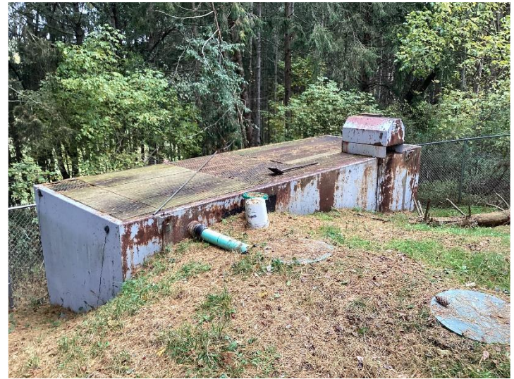
The existing sanitation packaging plant, which is in desperate need of replacement.
