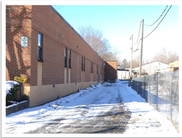
Existing Alderson Elementary at service drive with underground fuel tank below and a covered walk to old cafeteria building in distance.
