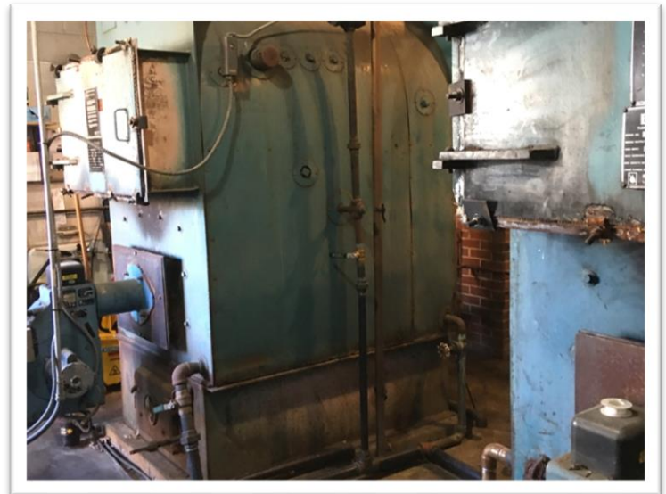
There is no air conditioning at the existing AES. Heat is provided by the propane fueled furnace at the main building.
