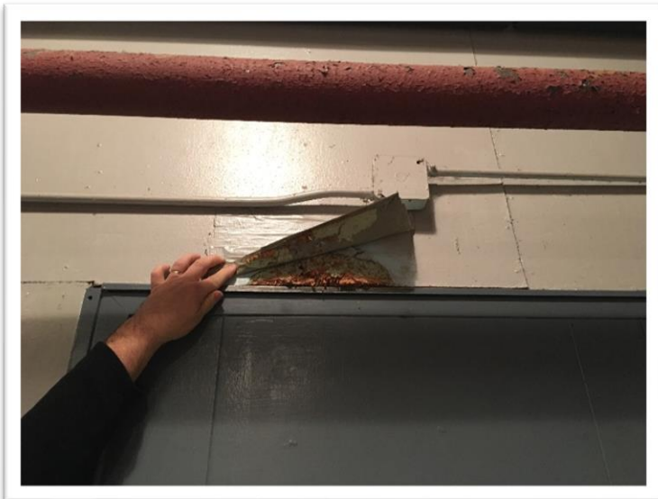
Existing AES cafeteria shows water damage in walls and exposed conduit and rusting exposed plumbing.
