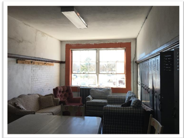
Second floor corridor in old high school showing ceiling height, window and wall condition.
