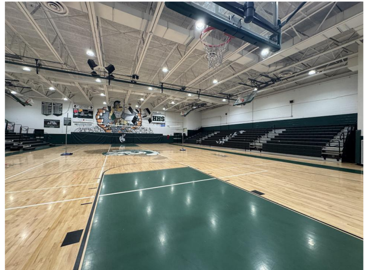
A new roof over the gym will prevent water penetration from damaging the floor.
