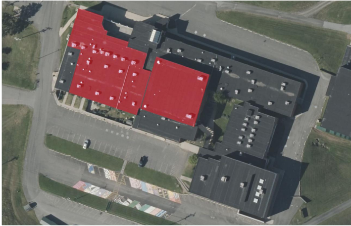
Highlighted area represents partial roof replacement at Hampshire High School.
