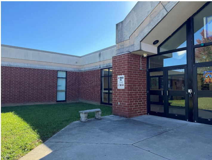
At Moorefield MS, an addition will be added to the left of the current entry for a new office and safe school vestibule.
