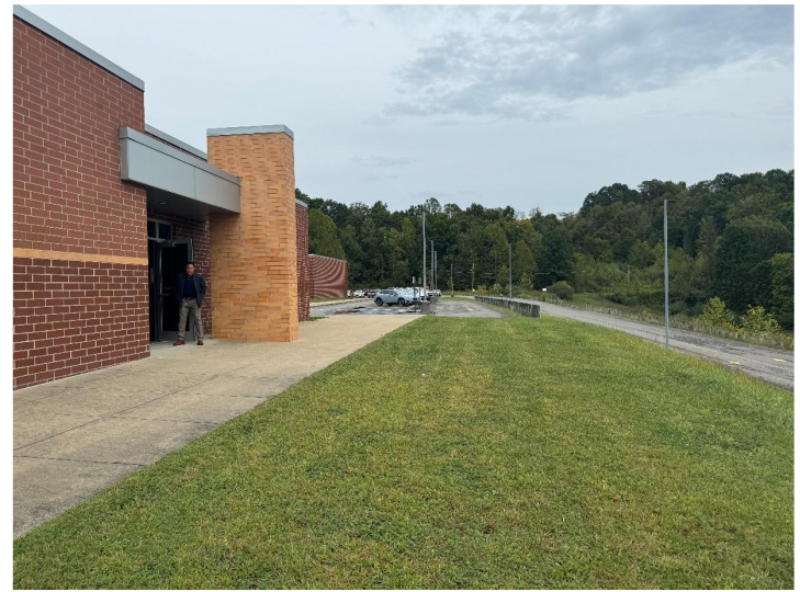
At Mountaineer MS, future PreK/ Kindergarten drop-off/pick up area is planned with renovations.
