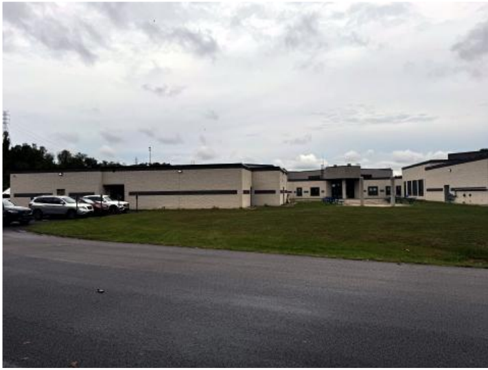
At RCB-HS, new CTC classrooms and a cafeteria addition will be constructed.
