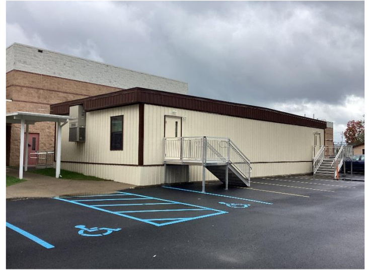
Modular classroom building that was added after the emergency closure of Norwood Elementary.
