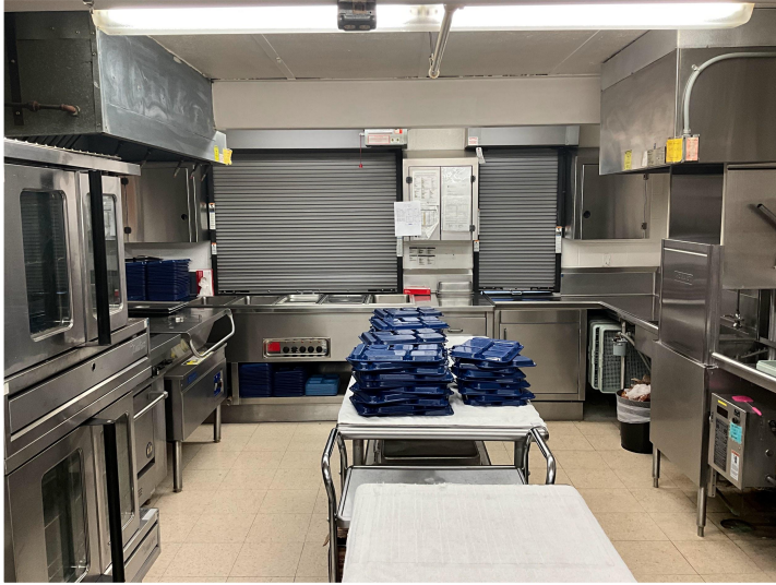
The kitchen is small and cramped, with food preparation and cleaning areas in close proximity, not complying with H&S codes.
