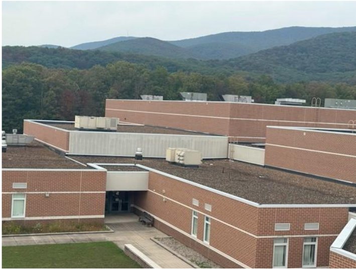
Scope includes replacement of two DOAS units serving most of the classroom and removal of the Ballast (gravel) roof.
