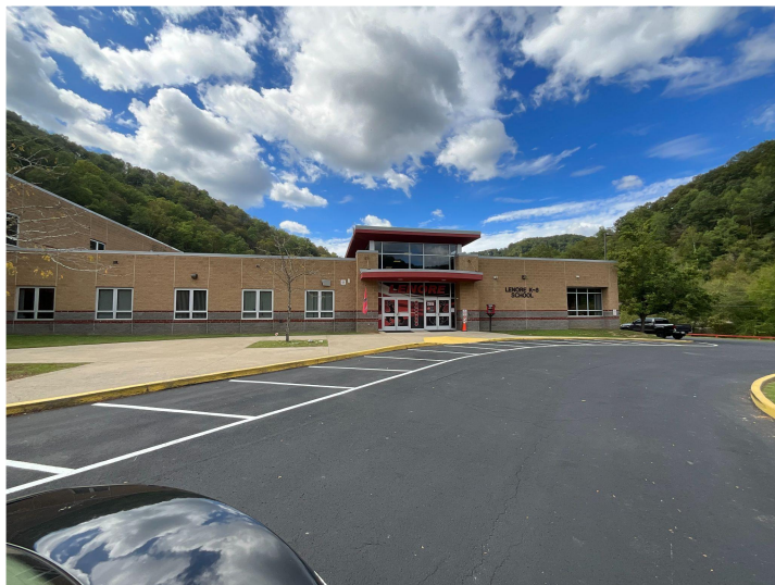
Lenore PK-8 was constructed in 2002. The HVAC system is constantly malfunctioning and causing health/safety issues.
