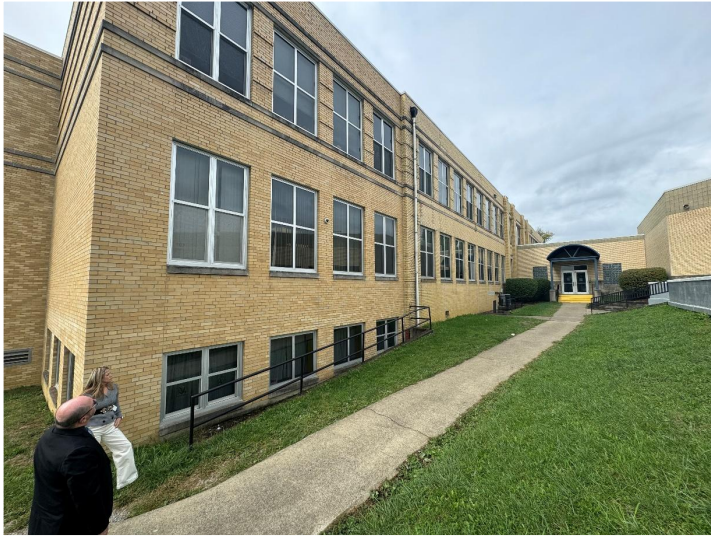
Suncrest MS's original three-story building was built in 1939 with a major addition in 1994.
