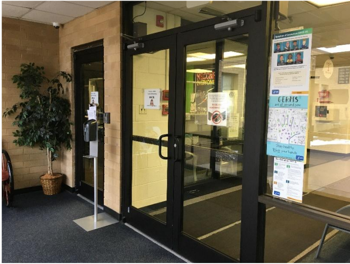
The vestibule mantrap renovation at MTEC involves adding a dividing wall which separates students and visitors.
