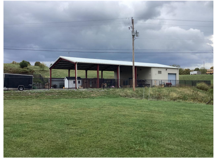
Existing warehouse shop space to be renovated and enclosed to better accommodate students and staff.
