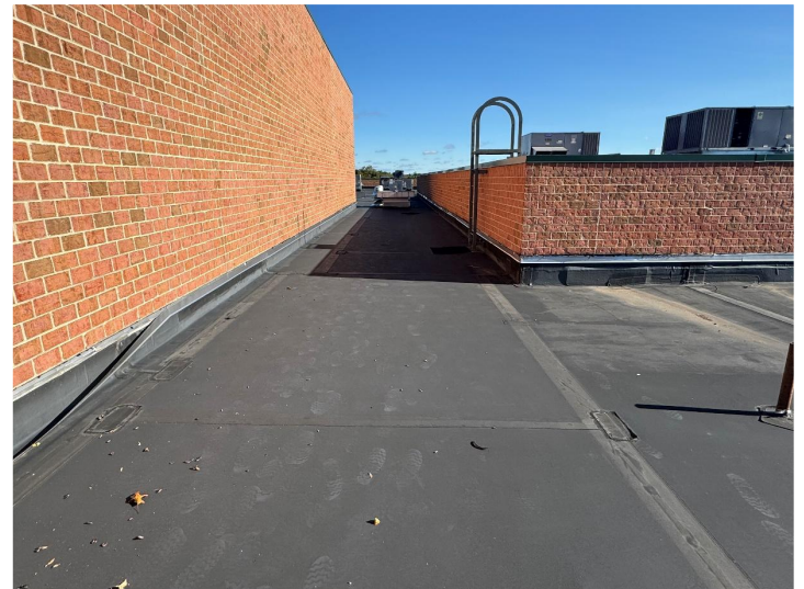
The roof overview at Warm Springs Middle
