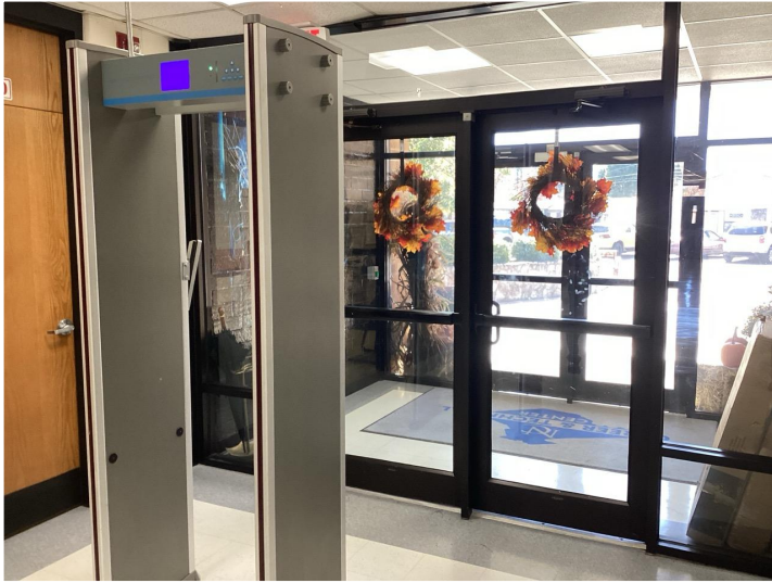
Existing main entrance to the facility to be renovated into a safe school entrance.
