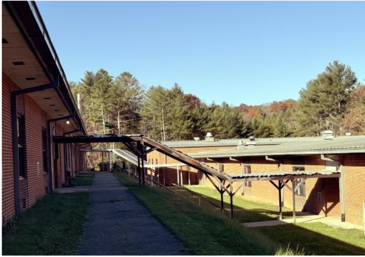
PCHS's project involves creating two enclosed corridors between the Main and CTC Annex Buildings.
