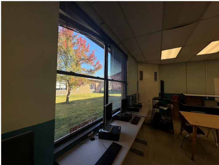
The scope involves replacement of windows and heat pumps in every room.
