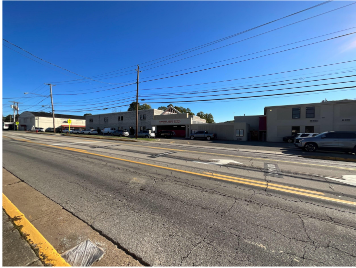
The existing, 74 year old school is outdated, undersized, and poses a health risk due to deterioration.
