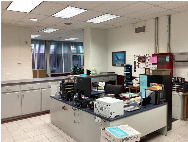
Existing administration area to be renovated into a new counseling and CIS suite.
