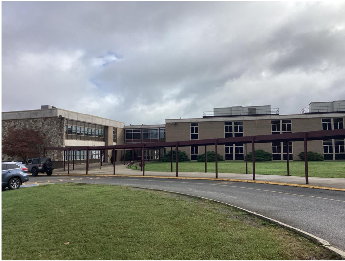
Proposed location of new administrative suite and safe school entrance at Woodrow Wilson High School.
