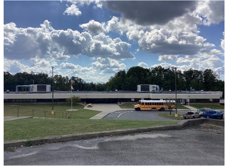
The adjacent Academy of Careers and Technology is supplied by the same water line.
