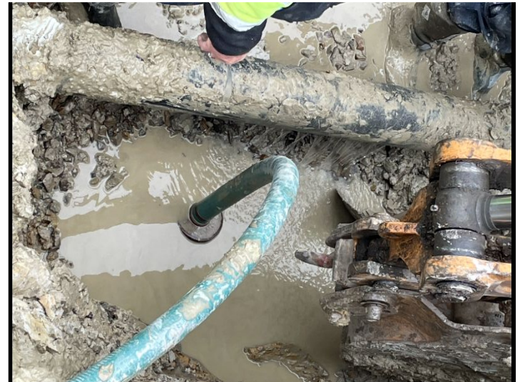
Water line repair at the Academy of Careers and Technology.
