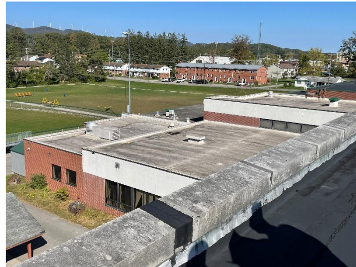
The area of school where sprayed insulation was placed.
