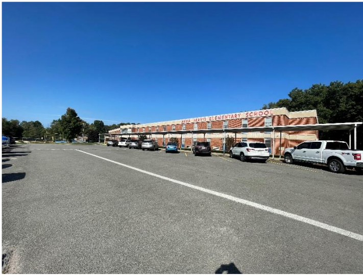
Current approach to school with covered walkway.
