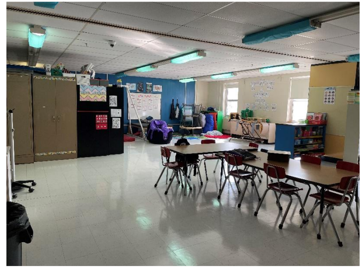
Typical classroom: this one is configured for special needs. HVAC are wall package units between windows.
