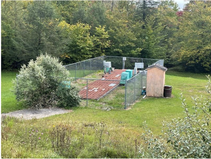
Sewage treatment plant is over the hill from school.
