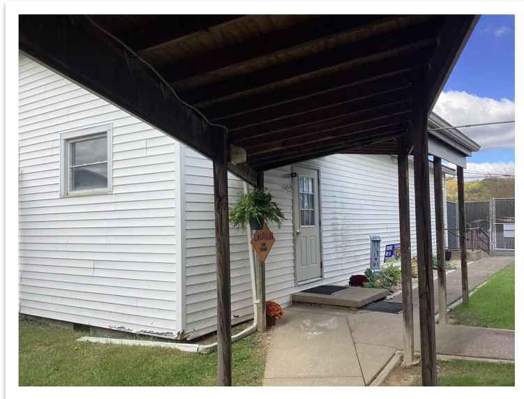
Outdated modular kindergarten classroom to be demolished.
