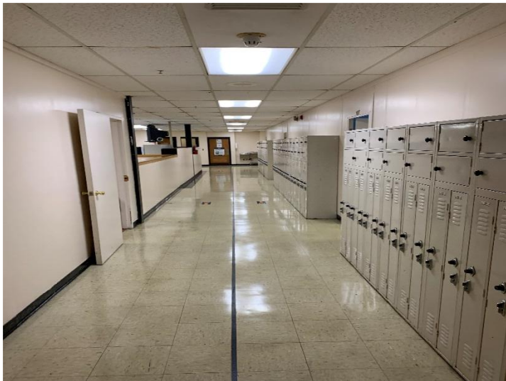
Project includes renovations to Buffalo MS to accommodate the additional students from Buffalo ES.
